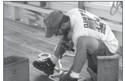
Up from Mystic, CT, caulker Chris Nelson drives cotton into the seams of the new quarterdeck
