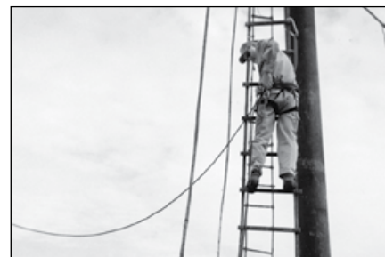
Bob Cannon climbing the shrouds to attach the triadic stay.
